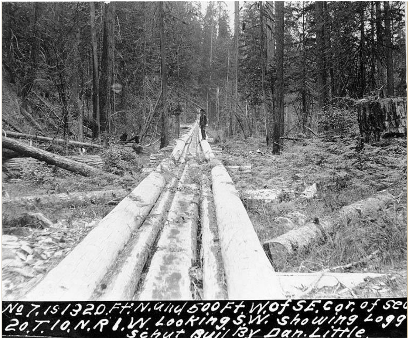
A log chute of long logs laid side by side, with a smoothed timber down the middle and a man standing at the far end, built by Dan Little near Kelso, Washington, about 1898. The handwritten caption on the original reads "showing logg schut built by Dan Little." Source: L. Heath, University of Washington Industries and Occupations Photographs Collection, via Wikimedia Commons (public domain).
